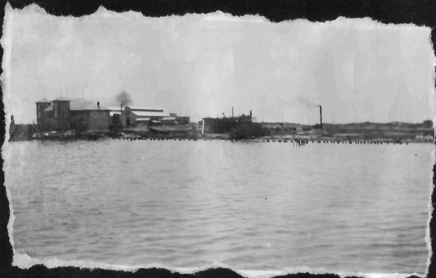
Building a Launch
