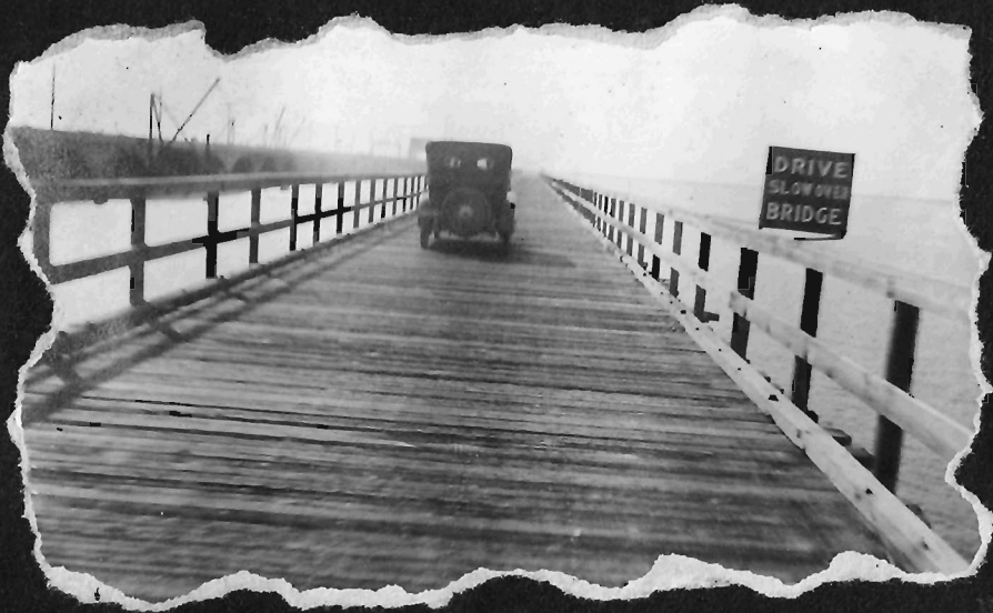
Showing the Nash crossing the Temporary Causeway, between the mainland of Texas and Galveston.
