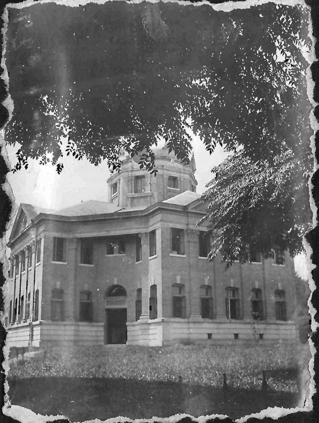
View of Courthouse
