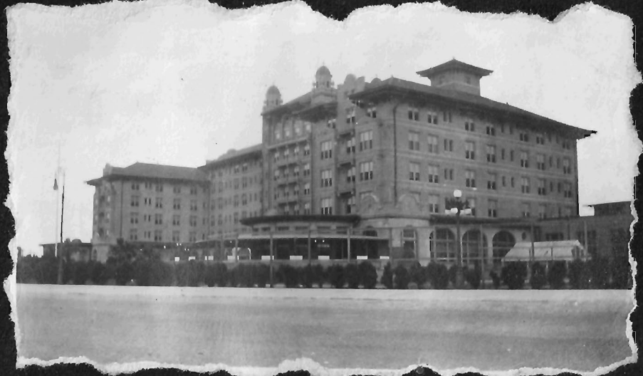
Galvez Hotel at Galveston costing $1,000,000 to build.
