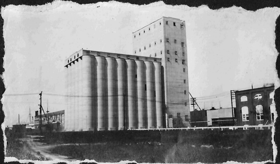
Elevator at Galveston having 48 bins and holding 1,000,000 bu. wheat.
